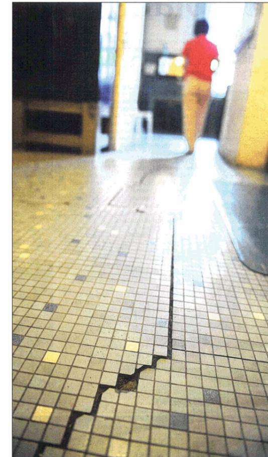
Cracks on the tiled floor of the church's sacristy, a room directly behind the altar of the sanctuary. The church, a national monument, has now called in engineers to study the extent of the damage and ways to restore the brick building. The church started noticing "quite a good number of cracks" after work began on the MRT Circle Line in 2003 and after the Singapore Management University had started work on its campus next door. ST PHOTOS: JOYCE FANG
